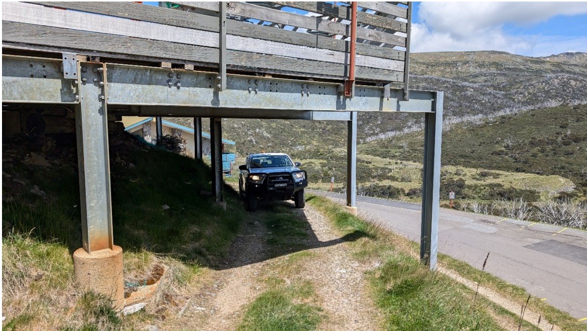
Figure 10: Insufficient clearance for larger vehicles via this route
